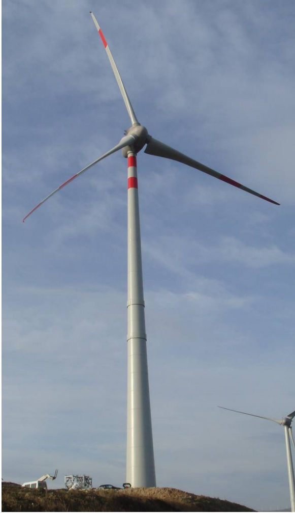
Figure 1: the 2MW wind turbine (ENERCON E-82)
