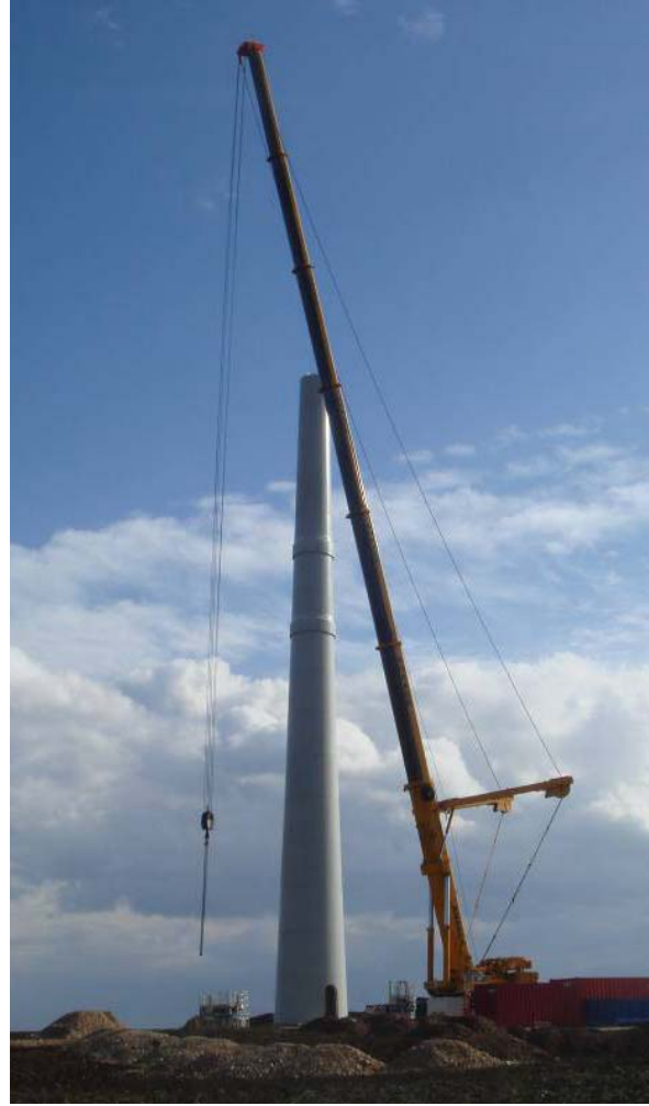
Figure 2: The concrete part and the first steel segment have been assembled
