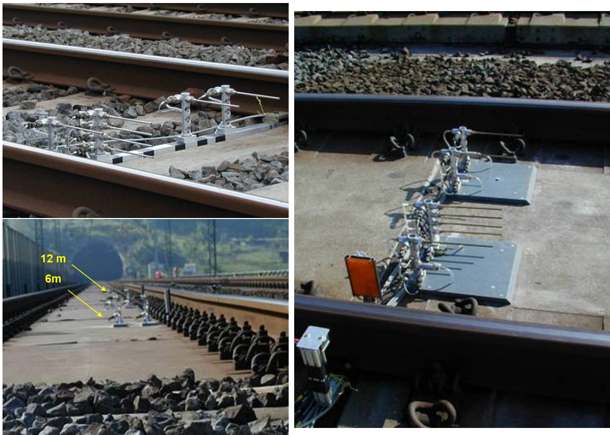
Figure 3: DBs Rakes of Pitot tubes installed on ballasted track and on slab track. The lower left shows the installations downstream of the interface between ballasted track and slab track.
