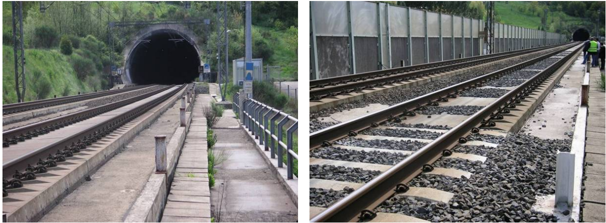
Figure 1: Track bed at the test site including slab track and ballasted track. Note the tunnel portal and the lateral wall along the left track.
