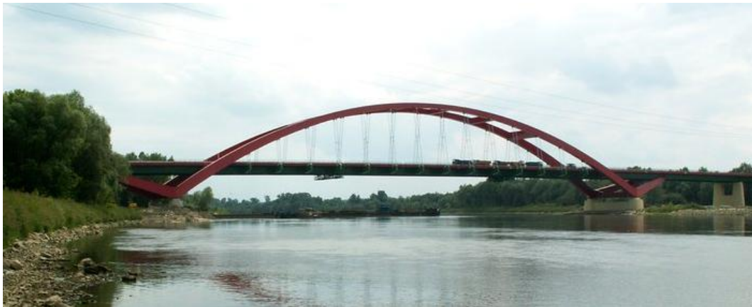
Figure 1: View of the arch bridge in Puławy.
