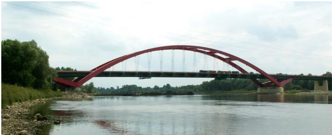
Figure 1: View of the arch bridge in Puławy.
