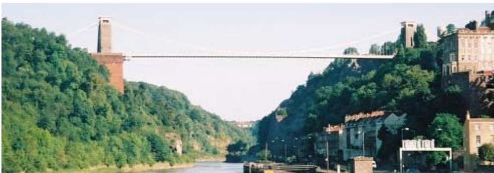
Figure 1: Picture of the Clifton Suspension Bridge.
